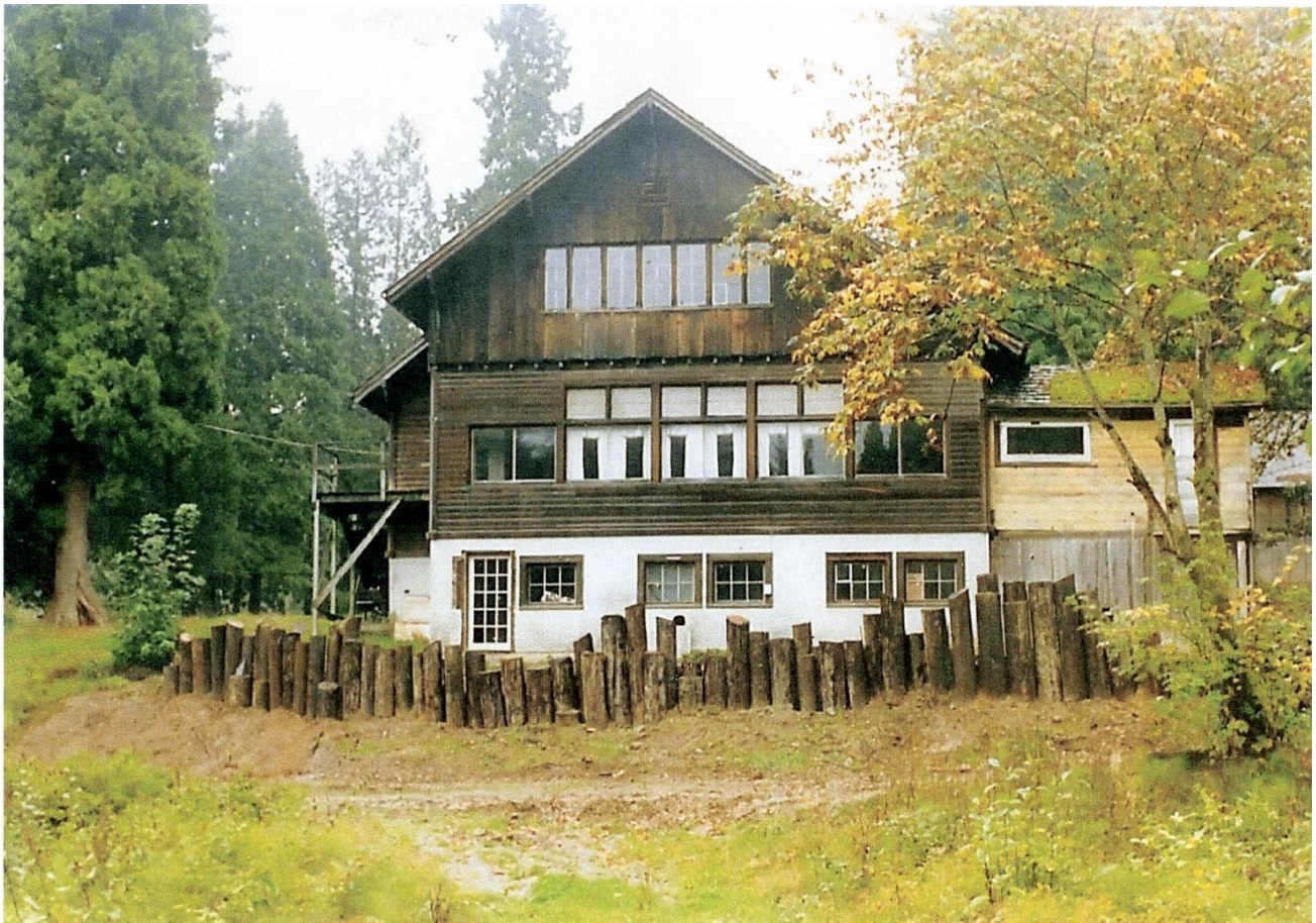
Figure 3 - Brooklake Community Center facing east, circa 1989. (Courtesy HSFW.)
