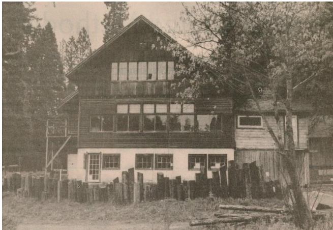
Figure 56 - Brooklake Community Center, facing east, April 1990. (Courtesy Rhonda Davis, Federal Way News .)
