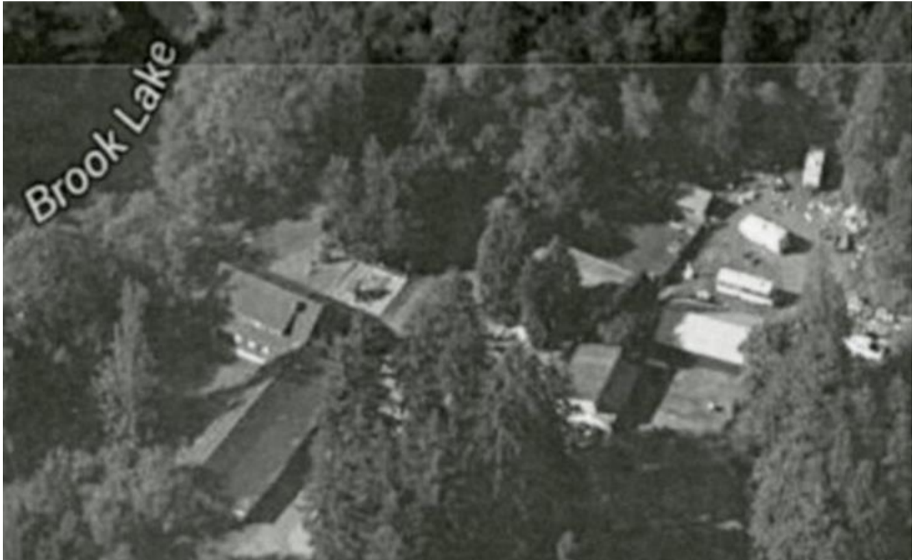
Figure 19 - Current Aerial Photo of Brooklake Community Center showing the Original Clubhouse Building, the Fair Building addition on the southeast of the original clubhouse, the Hall addition on the south of the original clubhouse, Outer Building 1 (OB1 about 80 feet in front of the Original Building), the Outer Building 2 (OB2 just to the northeast of OB1), and the mobile home west of OB2. (Courtesy Google Earth.)
