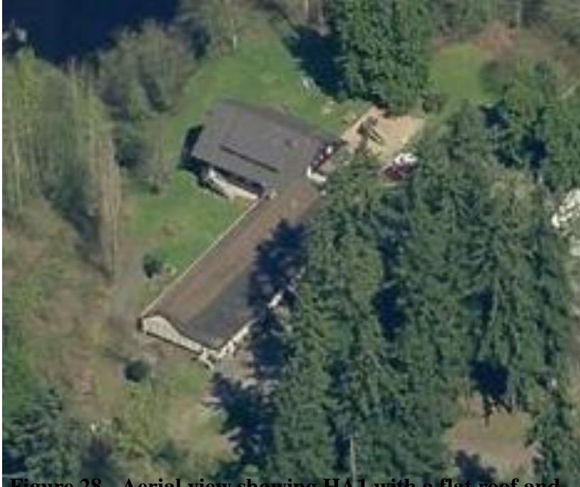
Figure 28 - Aerial view showing HA1 with a flat roof and HA2 with a sloped roof. (Courtesy Bing Maps.)
