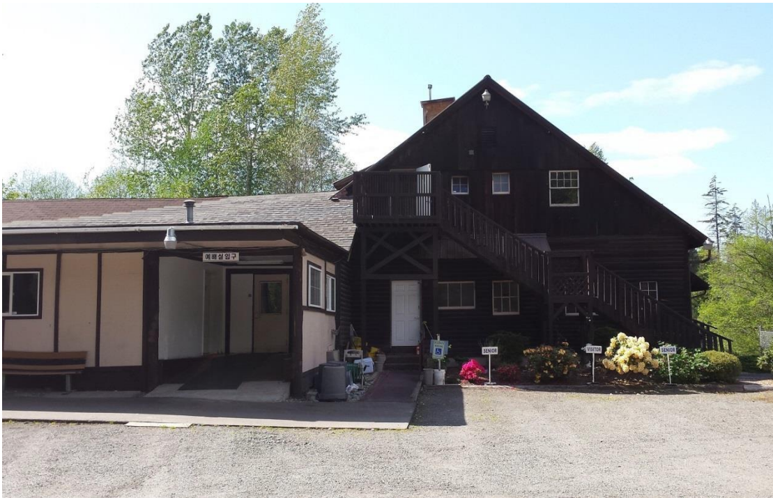
Figure 30 – The present entrance to the Brooklake Community Center, facing west, consisting of the conjoined Original Clubhouse Building, Fair Building and Hall. (Courtesy Karen Meador.)
