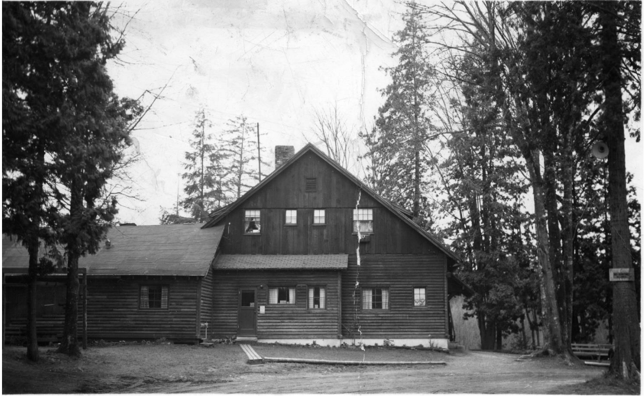
Figure 43 - Brooklake Community Center, with the Original Clubhouse Building and Fair Building addition, facing west, circa 1953. The date is based on the first known use of this particular photo, with the obvious visible crease in the middle, original on the cover of the Brooklake Woman's Club, Report on Community Service Contest, dated April 15, 1953. (Courtesy HSFw.)
