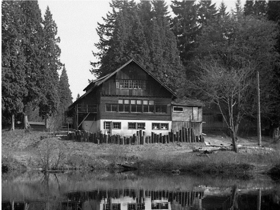
Figure 26 - Brooklake Clubhouse from rear, with clubhouse hall extension barely visible in background, facing east, circa 1953. (Courtesy HSFW.)
