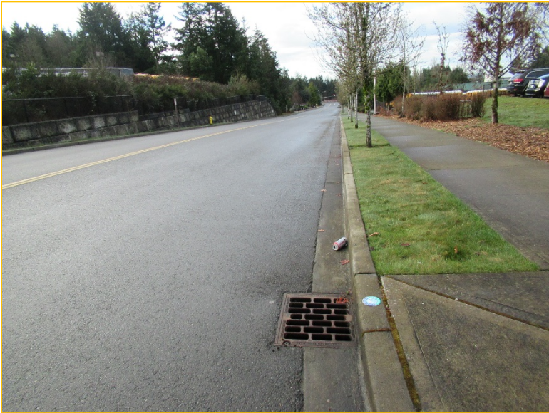
Photo 3B – Looking South – Flows continue south along the west side for 13 th Place South in a series of pipes and catch basins.
