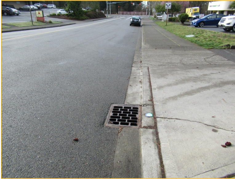
Photo 9B – Looking South – Flows continue south along the west side for 13 th Place South in a series of pipes and catch basins.
