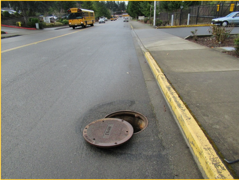
Photo 7B – Looking South – Flows continue south along the west side for 13 th Place South in a series of pipes and catch basins.
