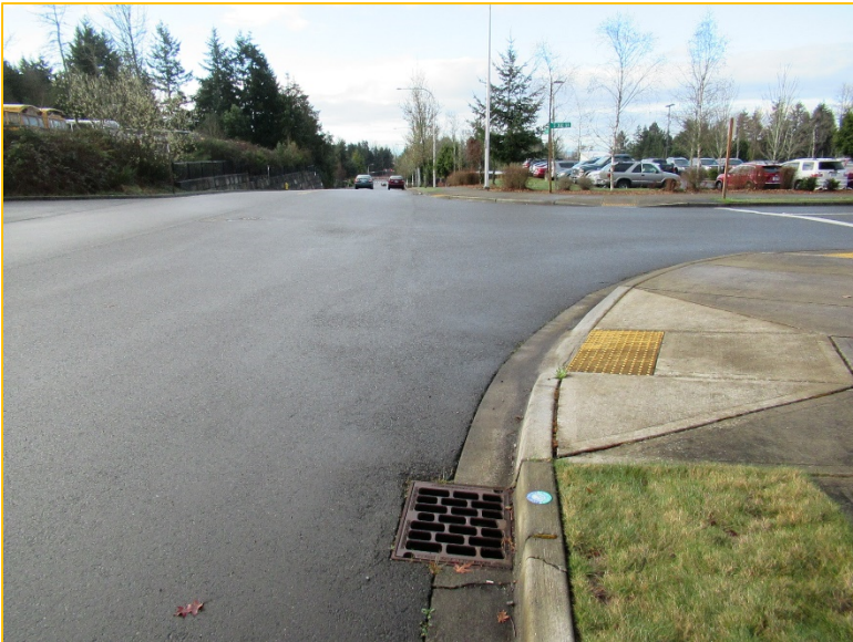
Photo 2B – Looking South – Flows enter the catch basin on the west side of 13 th Place South and is conveyed south across S 332 nd Street along the west side of 13 th Place South.
