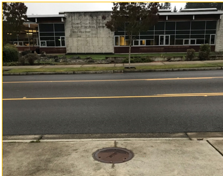
Photo 1C – Looking South – Runoff from the existing wetland west of the site enters the manhole above and continues south and southeast towards the parking lot of the Federal Way Public Schools Transportation Department.
