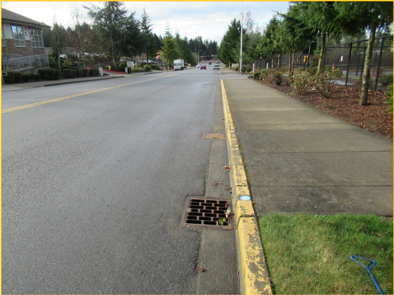
Photo 5B – Looking South – Flows continue south along the west side for 13 th Place South in a series of pipes and catch basins.
