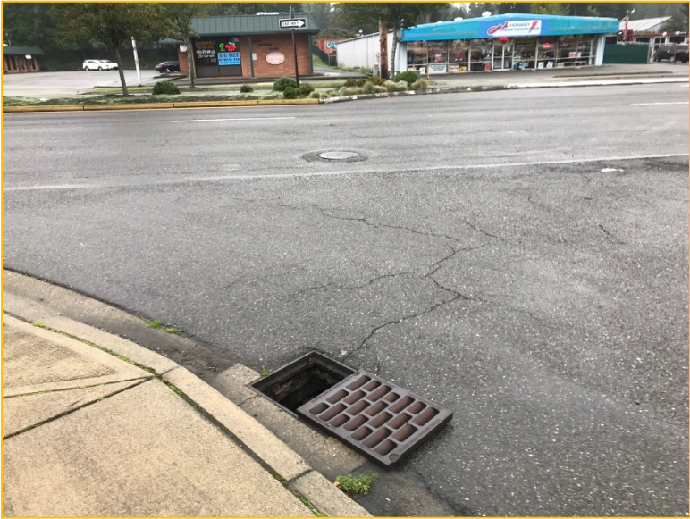
Photo 6A – Looking East – Flows are conveyed east from the catch basin to a manhole located in the southbound lanes of Pacific Highway South.
