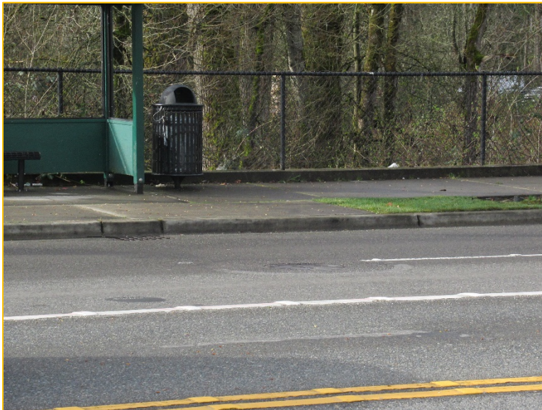
Photo 12B – Looking Southwest – Flows are conveyed southwest to a manhole located in the eastbound lanes of S 336 th Street.
