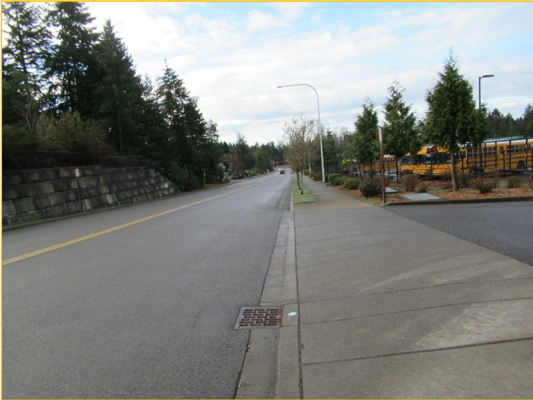
Photo 4B – Looking South – Flows continue south along the west side for 13 th Place South in a series of pipes and catch basins.
