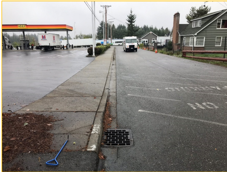
Photo 1A – Looking South – On-site flows from Basin A are captured in the catch basin and are conveyed south along the eastern side of 15 th Avenue S.
