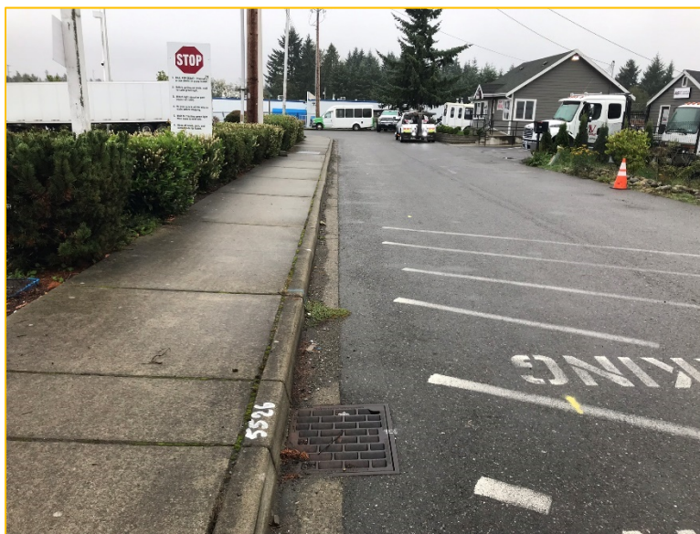
Photo 2A – Looking South – Flows continue south through a series of catch basins along the eastern side of 15 th Avenue S.
