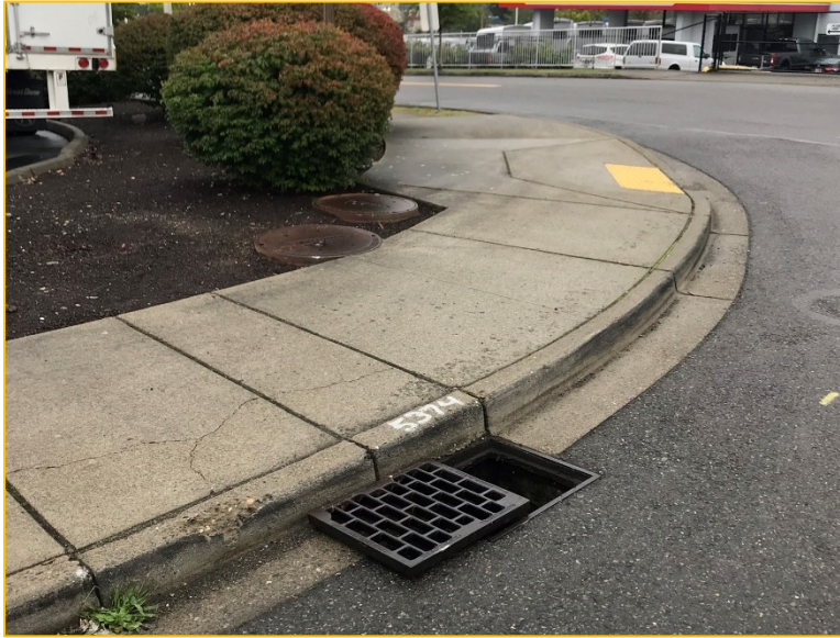
Photo 3A – Looking Southeast – Flows continue to the catch basin at the corner of 15 th Avenue S and S 332 nd Street. Runoff is then conveyed southeast to a series of catch basins located on the north side of S 332 nd Street.
