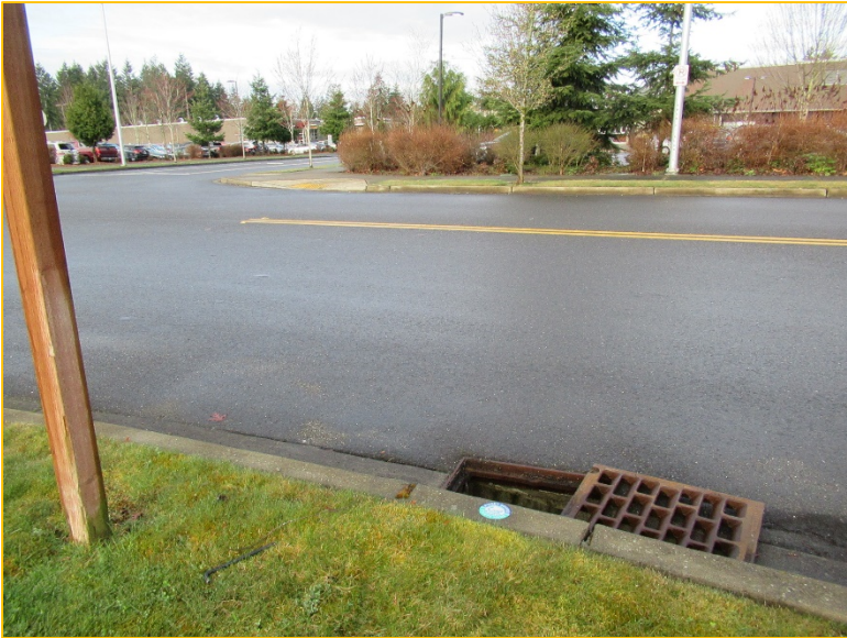
Photo 1B – Looking West – On-site flows flow south along 13 th Place South and enter the public storm system through a catch basin. Runoff is then conveyed west across 13 th Place South.
