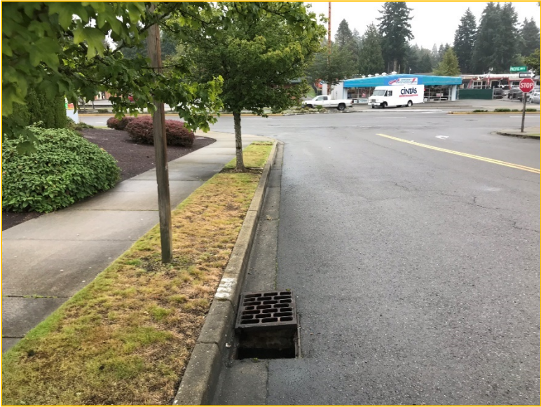
Photo 5A – Looking East – Flows are conveyed east along the north side of S 332 nd Street in a series of catch basins towards Pacific Highway S.
