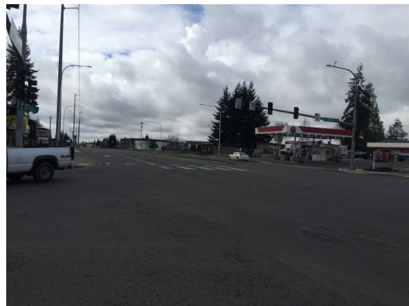
Intersection of Highway 99 and 304 th St
