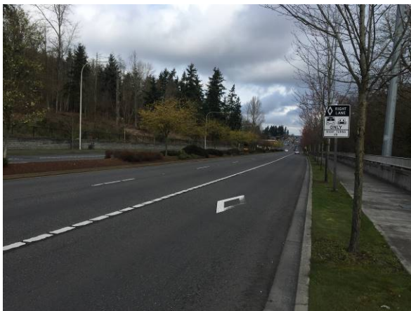
View north on Highway 99
