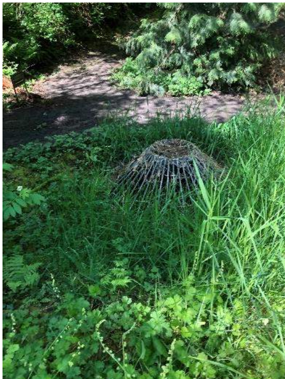
Photo 23 Catch basin/inlet between Asset ID # 21522 and ID # 21523 west of pool.
