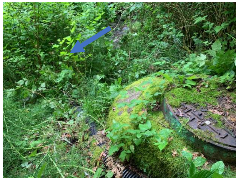
Photo 29. Manhole adjacent to creek.
