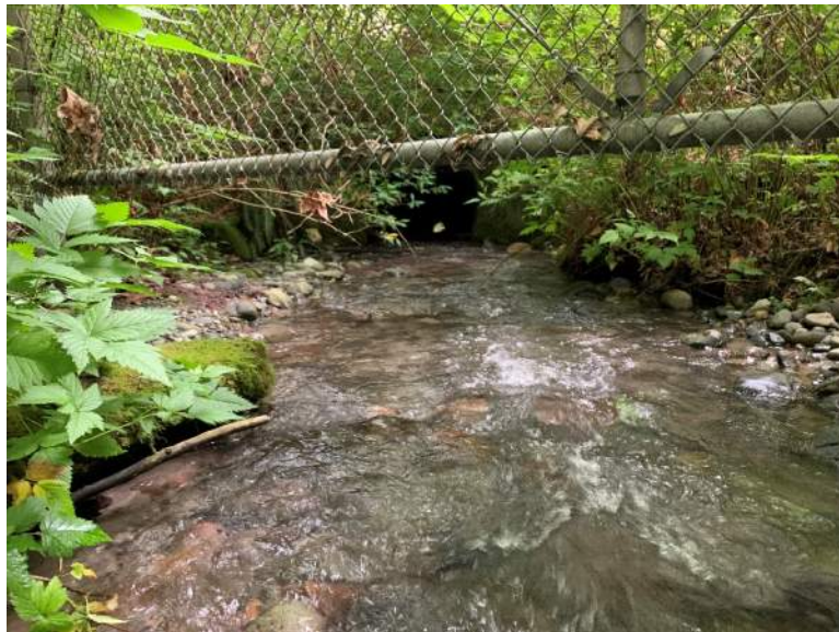
Photo 36: Transport reach to the culvert inlet at the water treatment plant.
