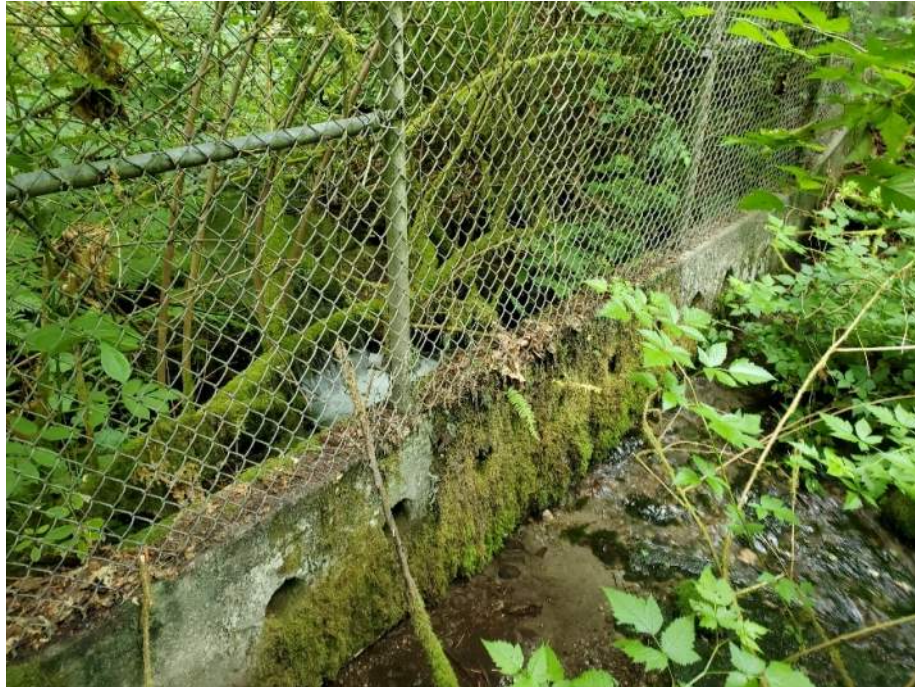
Photo 40: Concrete dam downstream of weir.
