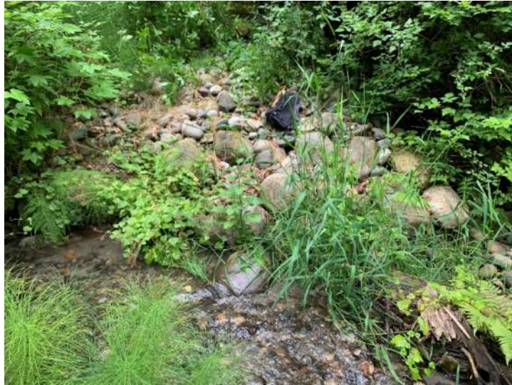
Photo 30. Large rock placed along left bank below CMP outlet.
