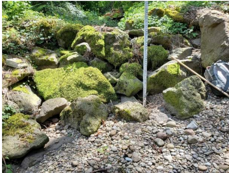
Photo 15: Lower artificial grade control downstream of residential area.
