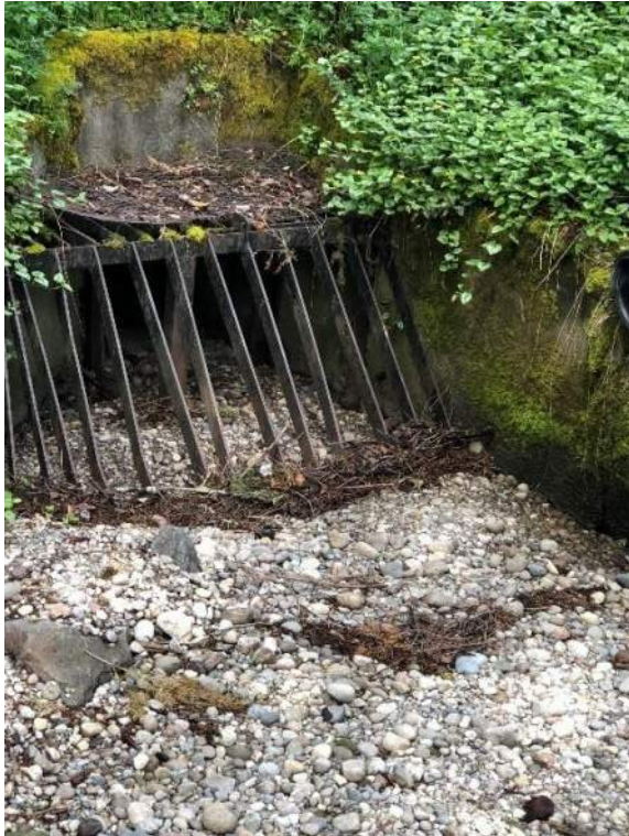
Photo 10 Marine Hills ID 19017 Inlet and steel grate cover.
