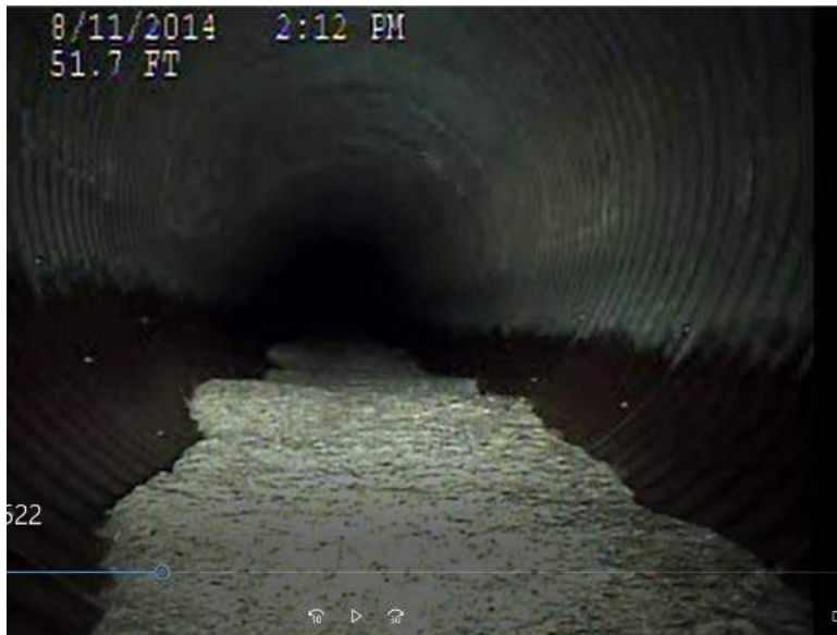
Photo 16 Typical concrete bottom liner for corrosion repair in CMP.
