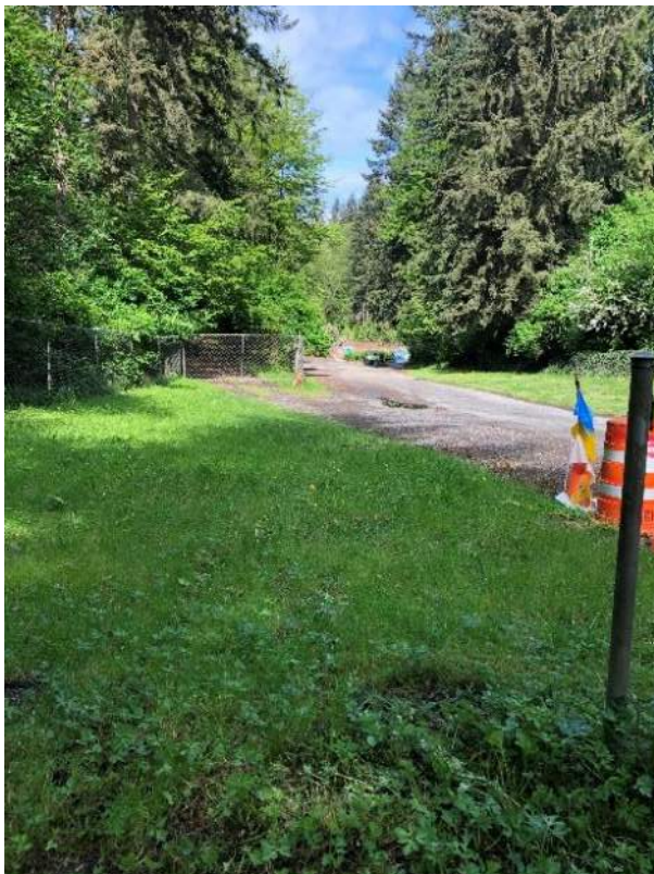
Photo 17 Asset ID 19021 looking west from inlet (adjacent to pool gate) along alignment towards pool and segment outlet.
