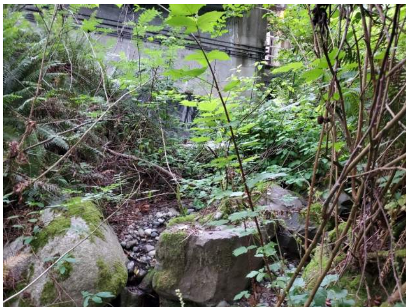
Photo 42. Treatment plant directly adjacent to right bank.
