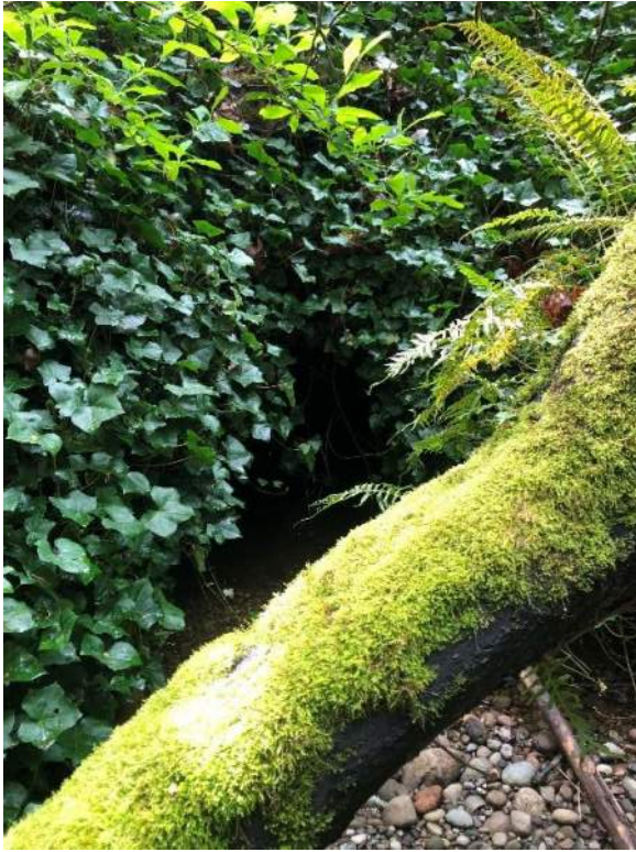
Photo 7 SR 509 42" CMP outlet.
