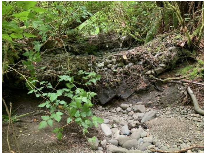
Photo 20: Last grade control series of gabions forming two 2-foot drops.
