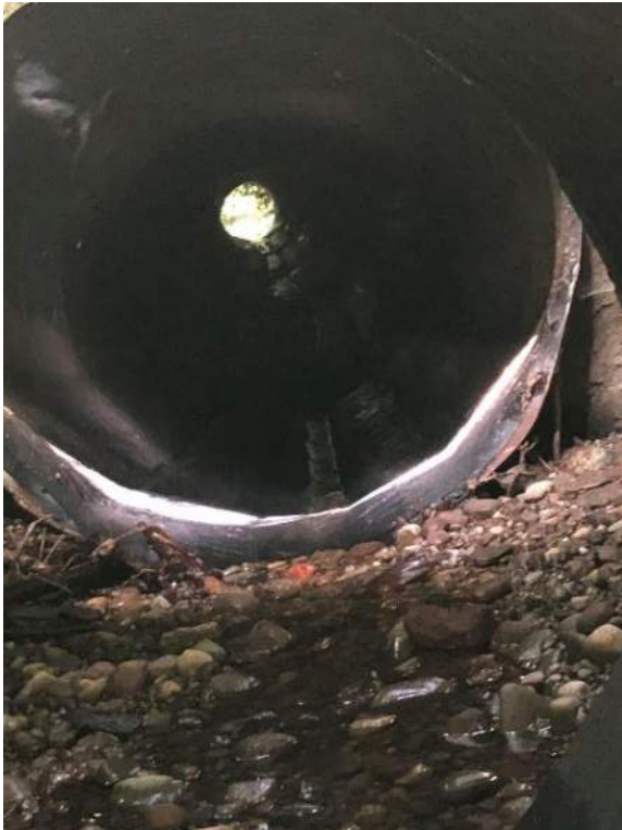
Photo 5 SR 509 View inside 36" CMP inlet looking at/thru 42" CMP.
