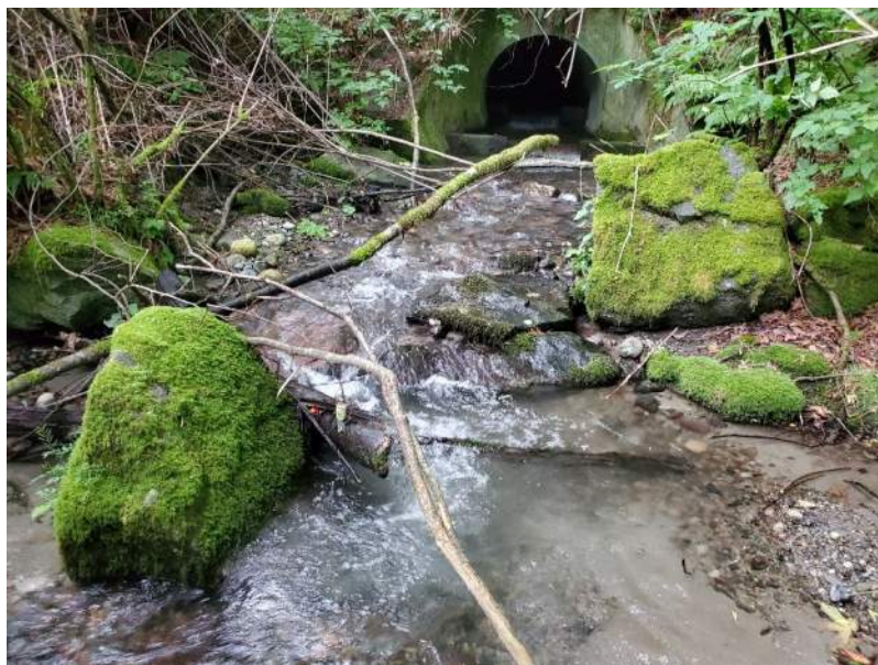
Photo 41. Baffled wastewater treatment plant culvert outlet.
