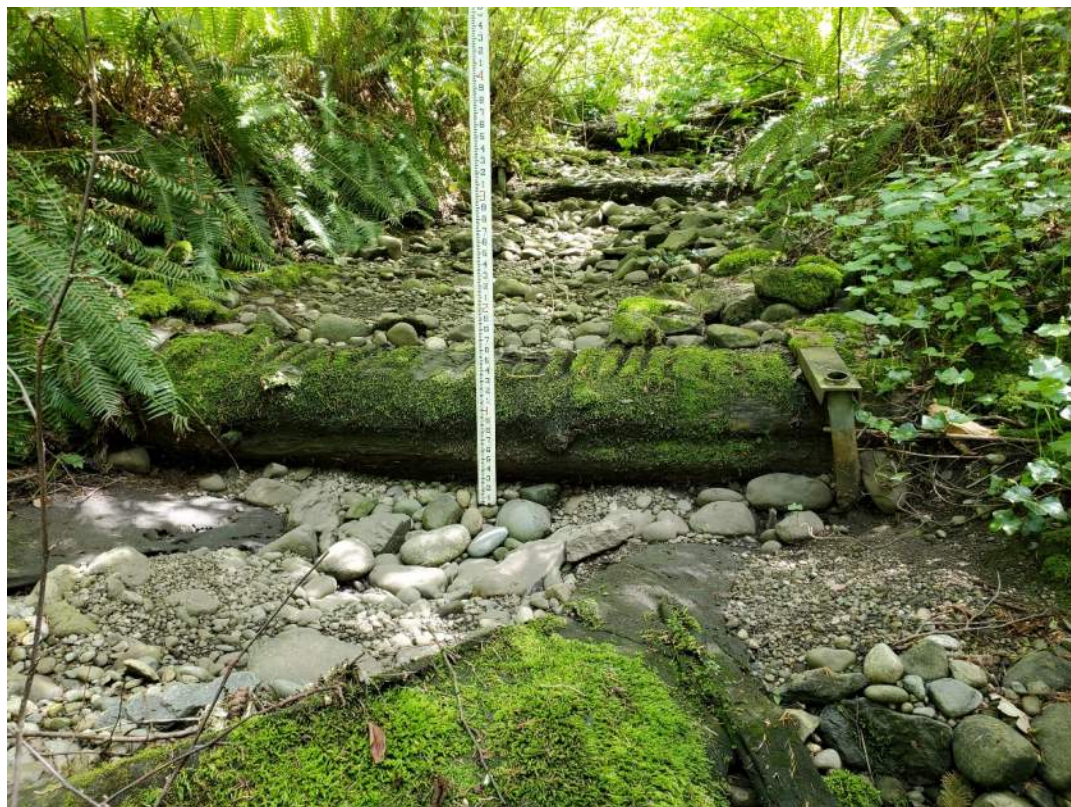
Photo 23. Series of log steps with moderate-sized scour pools and occasional exposed geotextile fabric.
