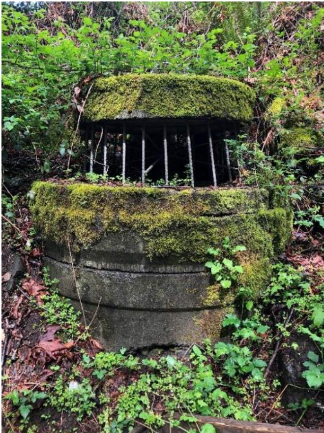
Photo 2 SR 509 overflow inlet weir.
