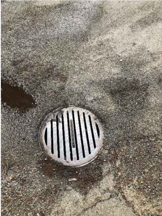
Photo 18 Asset ID 19021 to 21522 catch basin structure in pool west end of parking lot.
