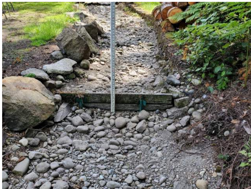
Photo 16. Additional channel modifications in downstream portion of Reach 2.
