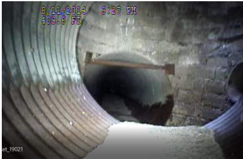
Photo 19 Asset # 19021 spring line drop into outlet manhole, approx. 2-foot drop.
