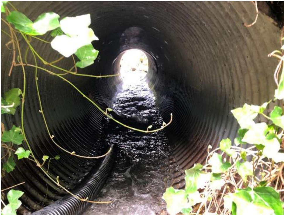
Photo 29 Redondo Shores Dr. S. inlet and CMP bore.
