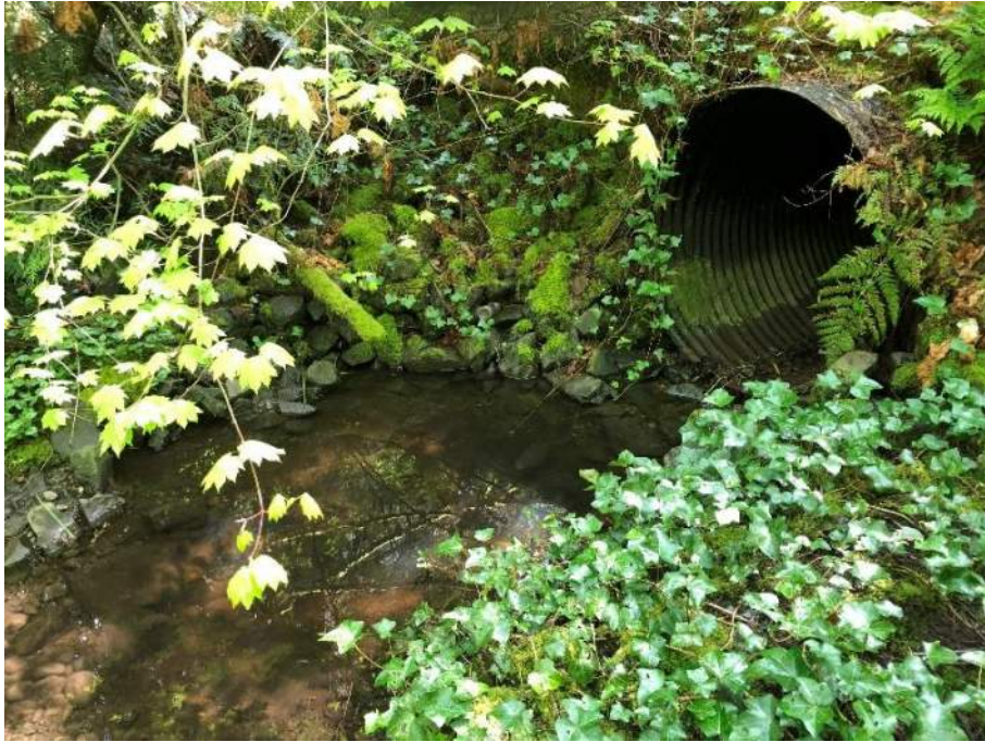
Photo 26 Outlet Asset ID 21523.
