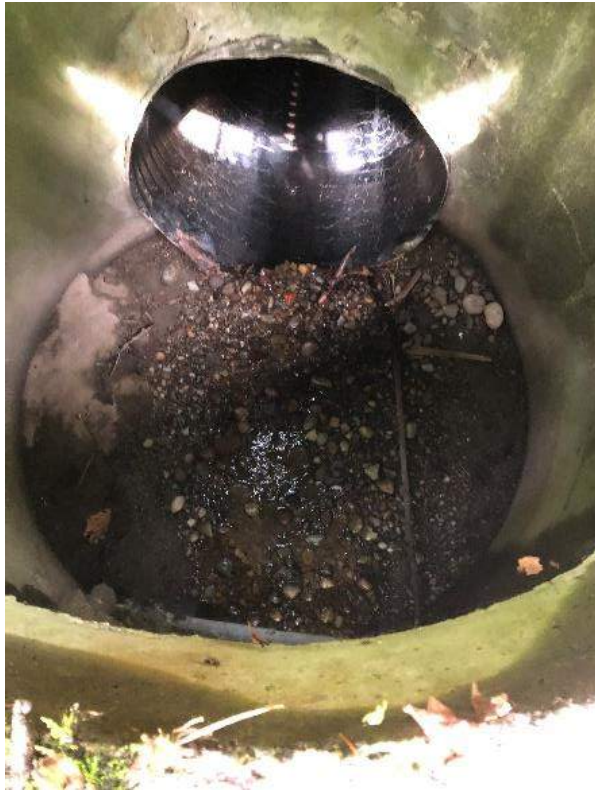
Photo 3 SR 509 View inside overflow weir and 42" CMP out flow.
