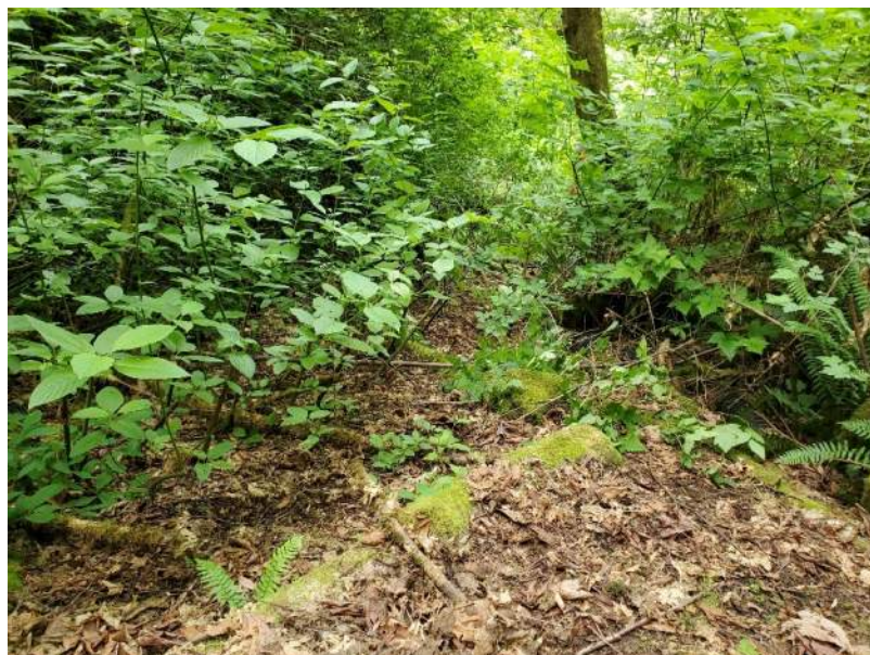
Photo 28. Cut vegetation along evenly-graded slope adjacent to CMP uphill of manhole.
