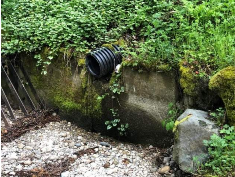
Photo 11 Marine Hills ID 19017 Headwall at inlet.
