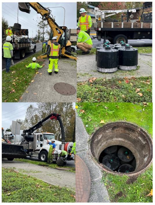
The Public Works Surface Water Management crew were out last week maintaining our stormwater vaults. Regular filter changes in these vaults helps ensure that harmful pollutants, like oil from vehicles, don't end up in our local waterways. Over 60 filters are maintained throughout the City, near major roads and highways. Residents can do their part in keeping our storm drains clean by remembering "Only Rain Down the Drain!"
