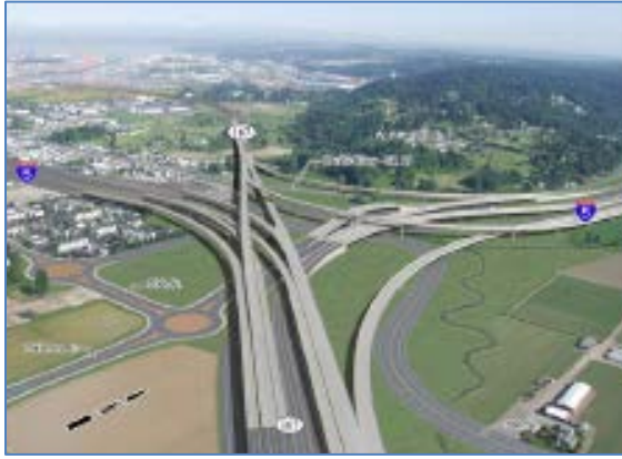
Figure 16: Artist's visualization of a possible design for an interchange connecting SR 167 and I-5 (looking northwest). Creek corridor at lower right is the re-channelized and restored Surprise Lake tributary (WSDOT, SR 167 FEIS)
