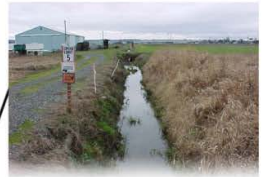
Existing Surprise Lake Drain
